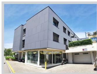
BIPV Facade Zurich, Switzerland
